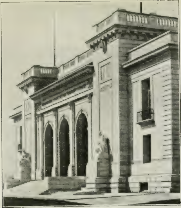
BUILDING A NEW-YORK, 5 e AV.
